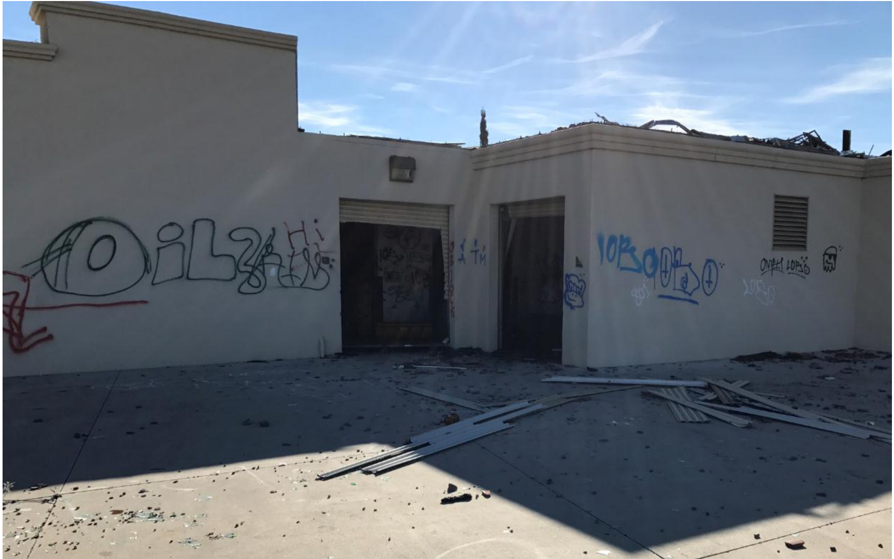
View of cart barn (basement) of former clubhouse, looking east.
